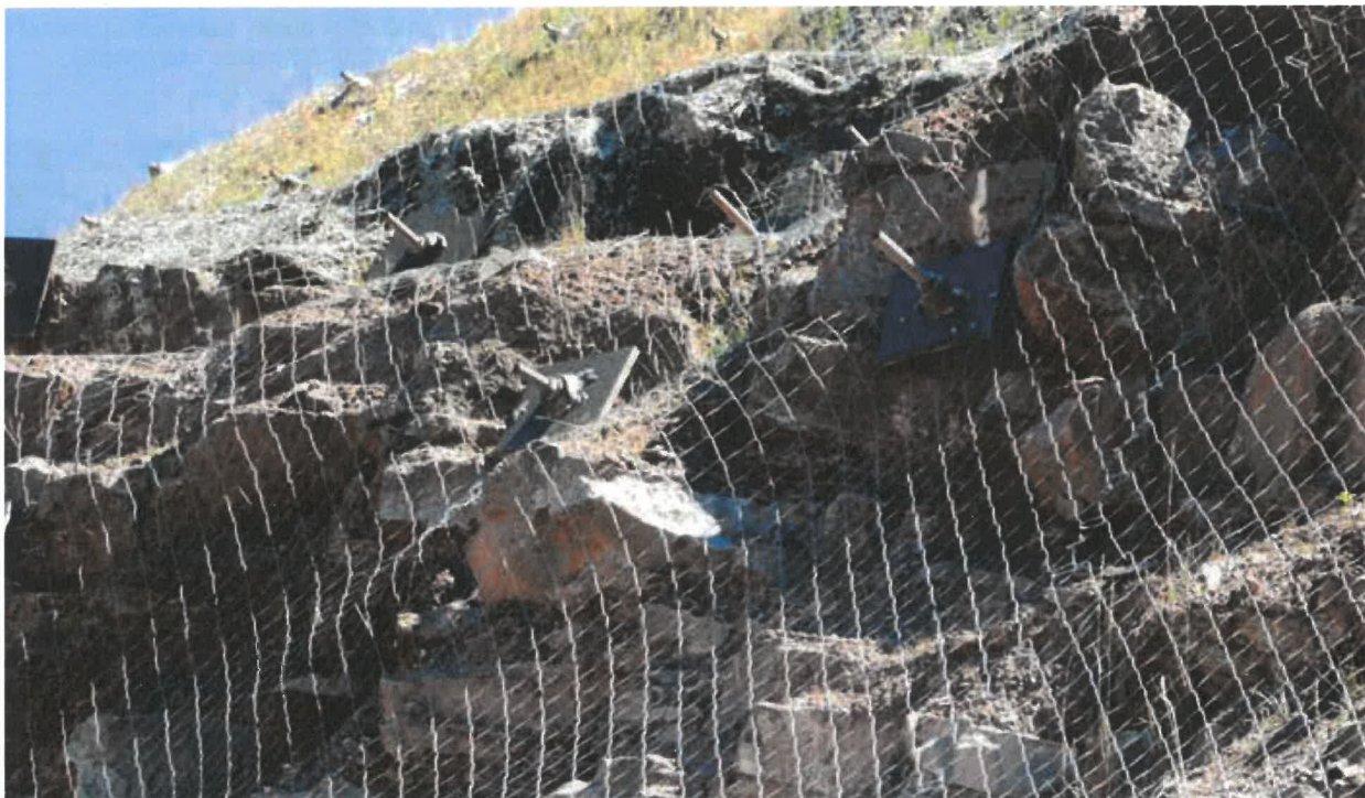
GEW® Rock Bolts & DELTAX® – Installation at Heads of The Valley Road Improvement Scheme, A465 South Wales
